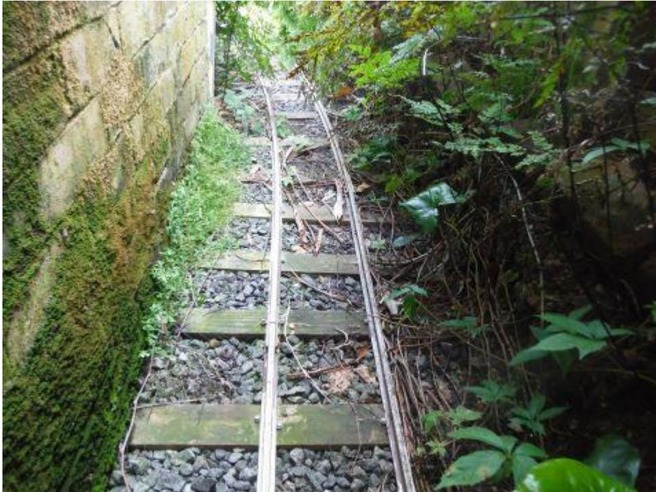
A section of ballasted track on an otherwise lightly built line. The long sleepers and a tightly packed bed of sharp stone keep the track in place while still allowing rain water to pass beneath,
